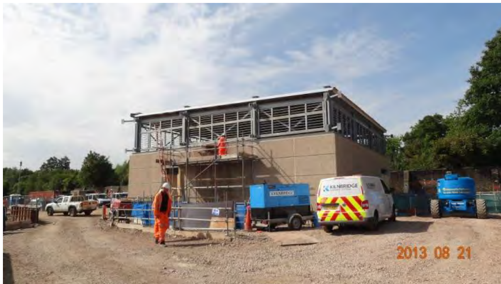
Figure 5.6 Tunnel Head House under Construction
