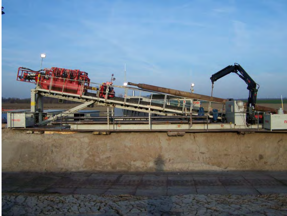
Figure 5.7: Horizontal Drilling Rig
