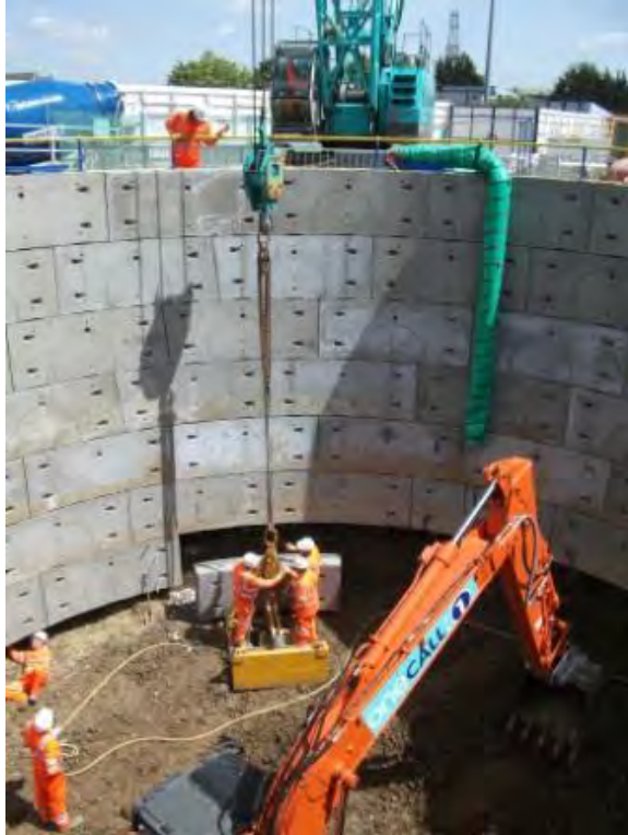
Figure 5.4: Tunnel shaft in construction (National Grid: London Tunnels)
